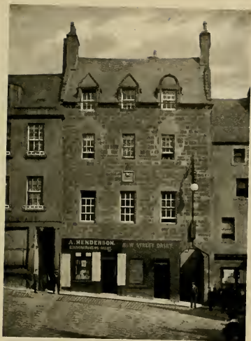
DARNLEY HOUSE, BOW STREET.
